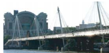
写真21, Hungerford Bridge, London, UK. (2002)
