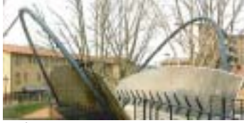
写真26,Rotherhithe Tunnel Bridge, London,UK.(1998)
