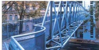
写真9, Koliste Footbridge, Brno, Czech Republic. (1998)
