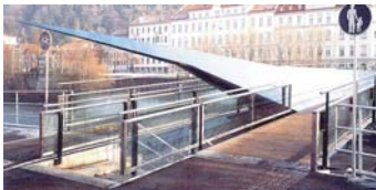
写真12, Footbridge Over The River Mur, Graz, Austria. (1992)
