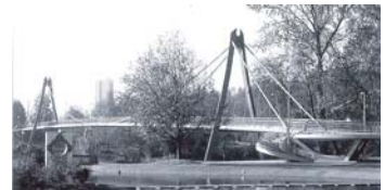
写真19, Willamette River Pedestrian Bridge, Eugene, USA. (1999)
