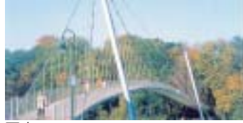
写真36,Pedestrian Bridge over The Weser River,Minden,Germany.(1996)
