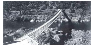
写真17, Sacramento River Trail Pedestrian Bridge, Redding, USA. (1990)
