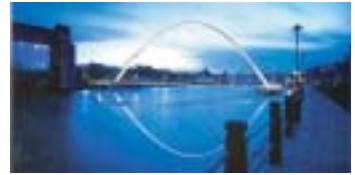
写真43,Gateshead Millennium Bridge, Gateshead,UK.(2001)
