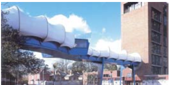
写真4, Plasht School Footbridge, London, UK. (2000)
