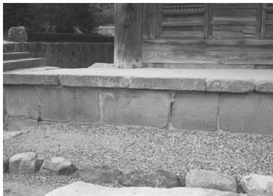
Photo 6. Foundation of Tondo-sa
