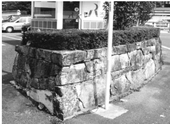
Photo 9. Restored stone wall
