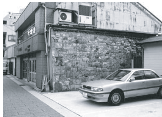
Photo 5. Existing fire wall
