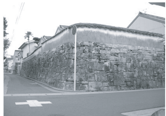
Photo 3. Existing stone wall with round corner
